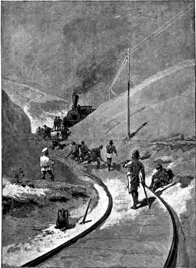
CLEARING AWAY THE SAND
